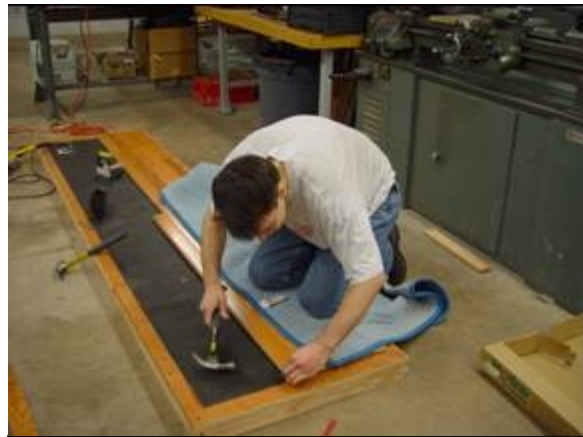
Figure 5: Construction of Profile 10, Oak Flooring
